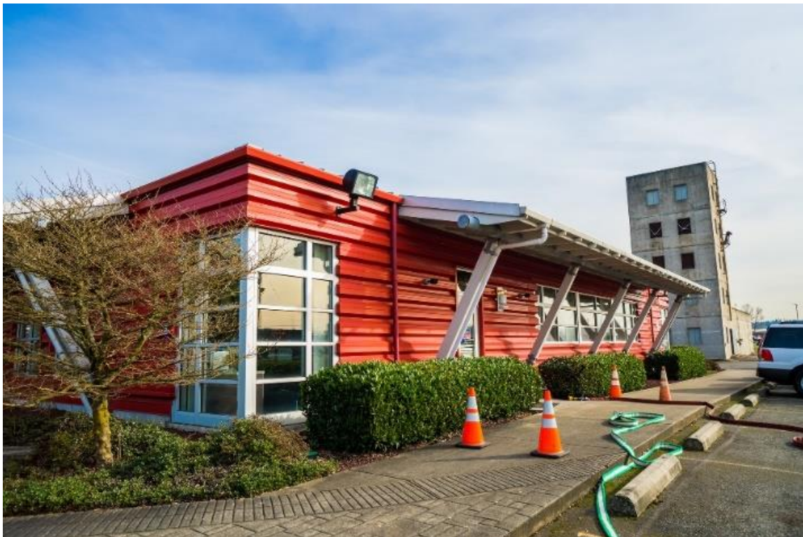
Tacoma Fire Training Center
